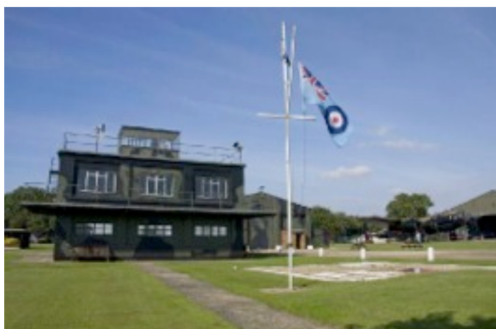
East Kirkby Control Tower
